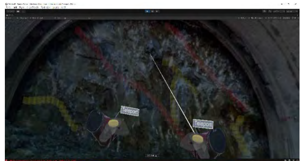
Photo 5 VR system user's viewpoint after the cracks were colored.
