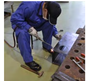
Figure 4. Welding the steel plates
