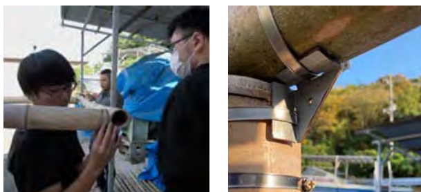
Figure 8. Assembling the bamboo house
